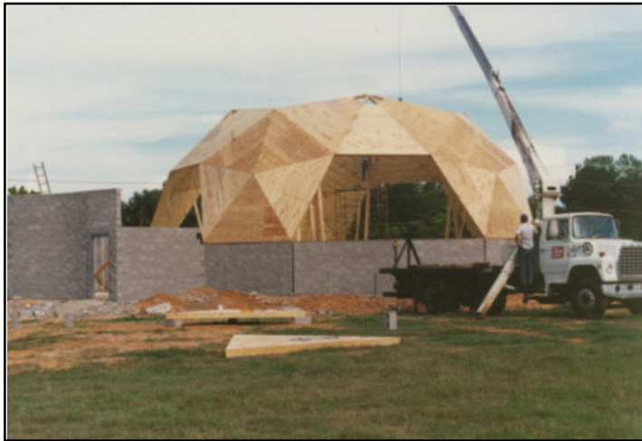
Image 4.8: The library's original dome (under construction above) was intended to be the first of three such structures. In order to serve a growing community the library will need to physically expand its facilities proportionate to the City's population growth.
