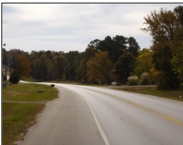
Image 7.7: Highways within the ETJ which are maintained by TxDOT or the County are frequently kept in excellent condition; however, some problems were observed on shoulders which are not curbed.
