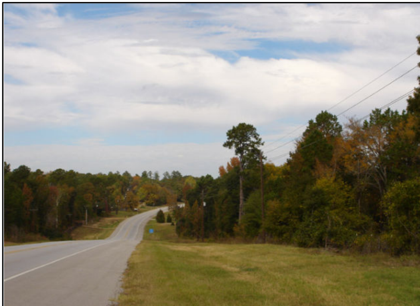
Image 7.3: Open ditches such as these found on State Highway 110 South provide drainage control throughout most parts of the ETJ.
